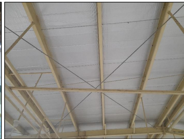
Roof bracing
