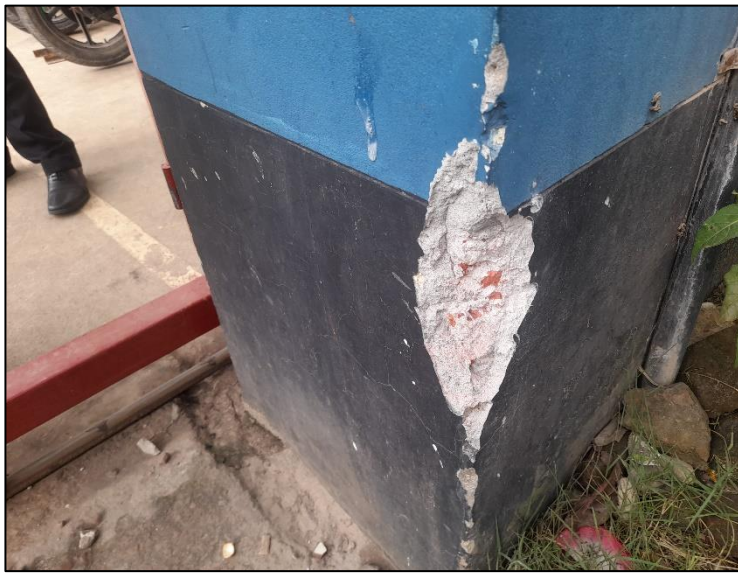
Brick aggregate (Security Guard room)
