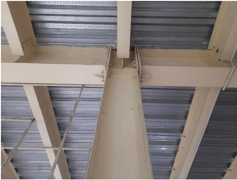
Beam-Column frame system
