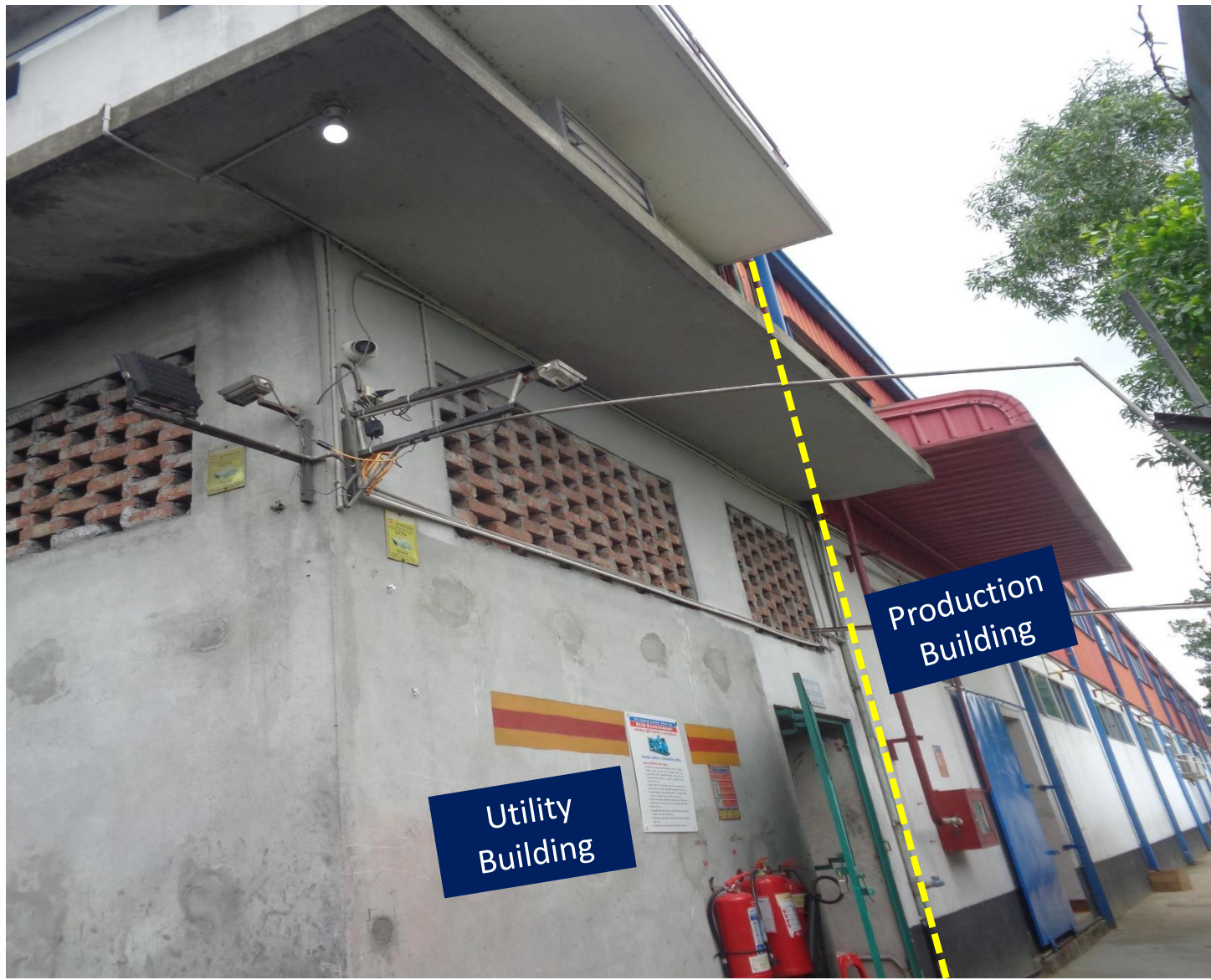
Utility Building & Production Building Structurally Separated with Expansion Gap
