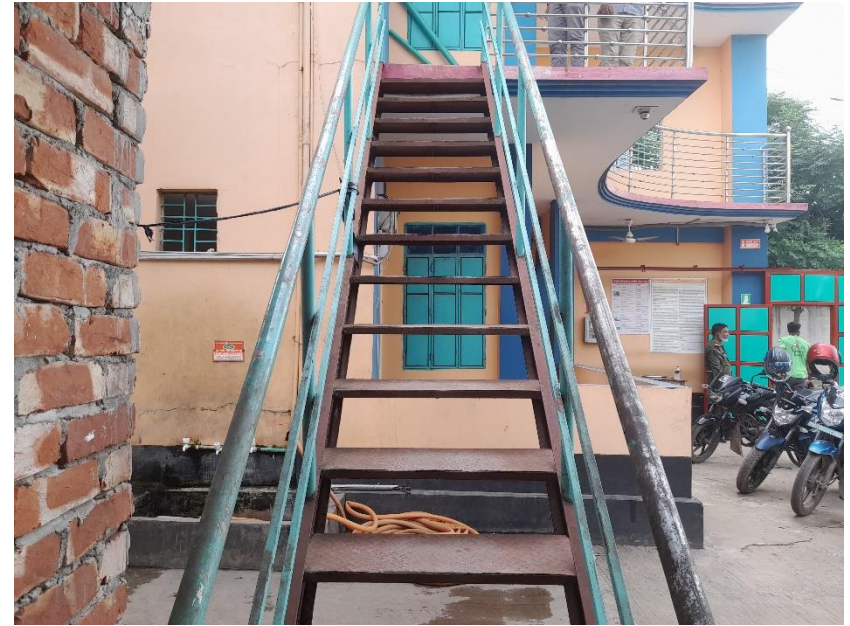
Non-engineered steel stair
