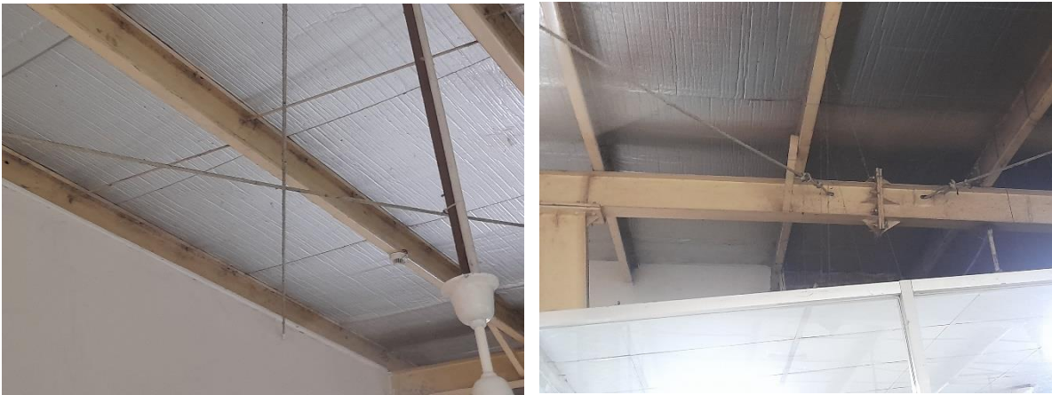
Horizontal Bracing
