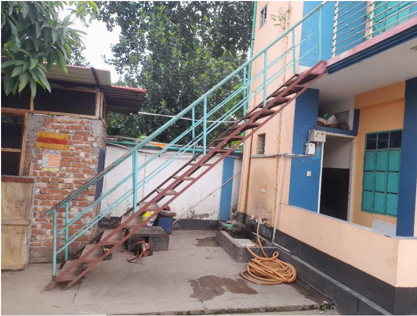
Non-engineered steel stair
