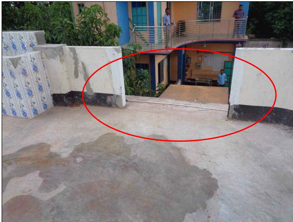
Opening at parapet wall
