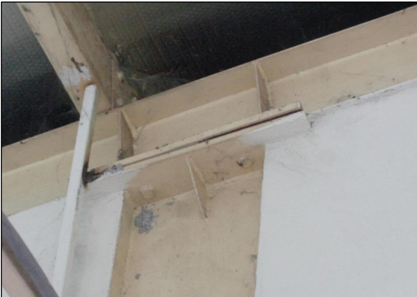
Significant gap in steel connection plates in different location
