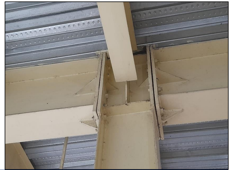
Significant gap in steel connection plates in different location
