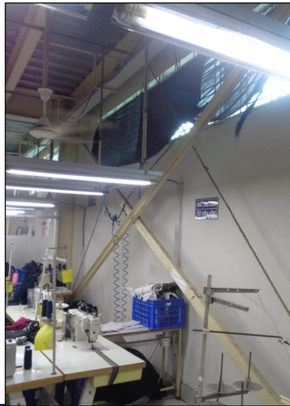
Roof & wall bracing provided
