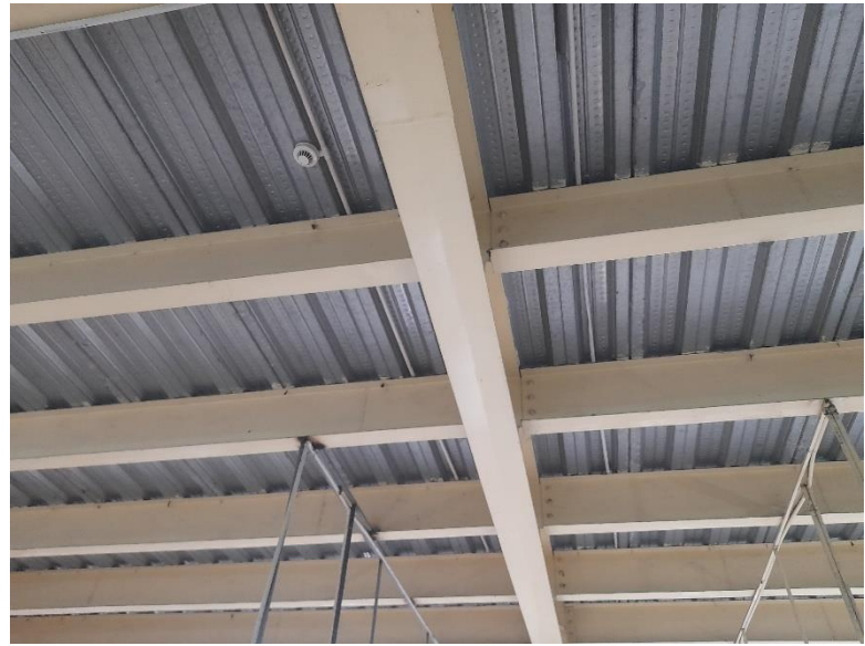
Main Beam to Sub-beam connection
