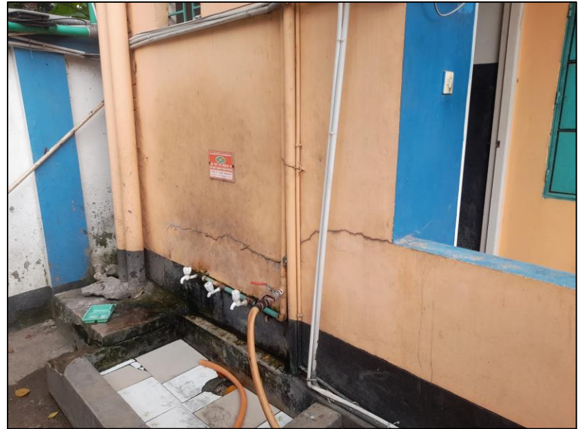
Cracks on masonry walls
