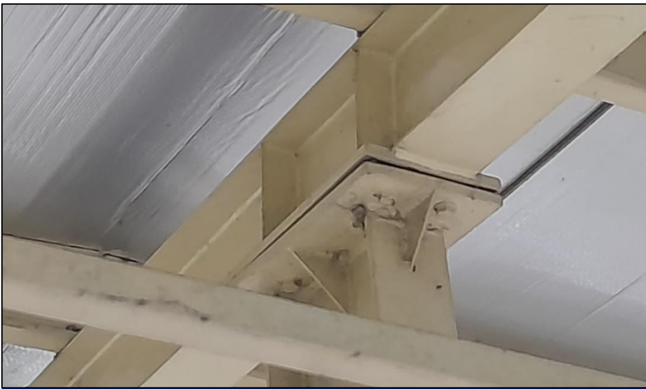
Significant gap in steel connection plates in different location
