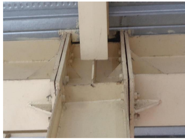
Connection Type Bolted
