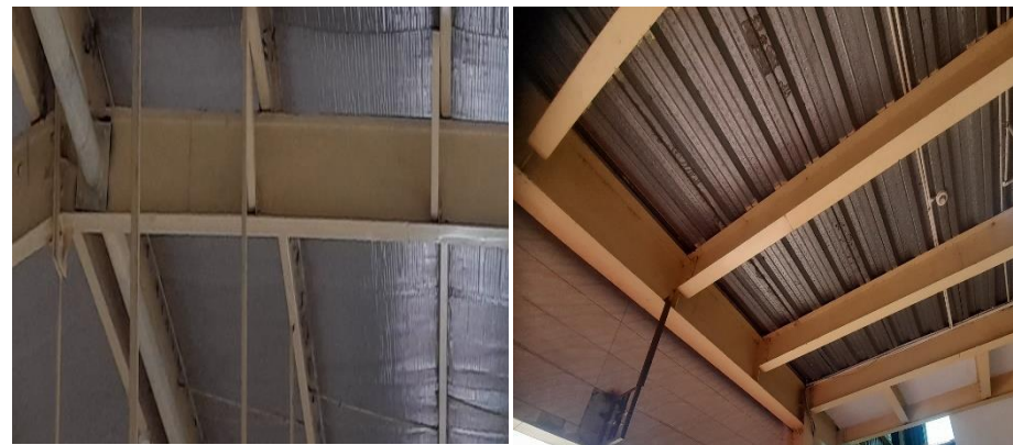
Rafter & Deck Slab
