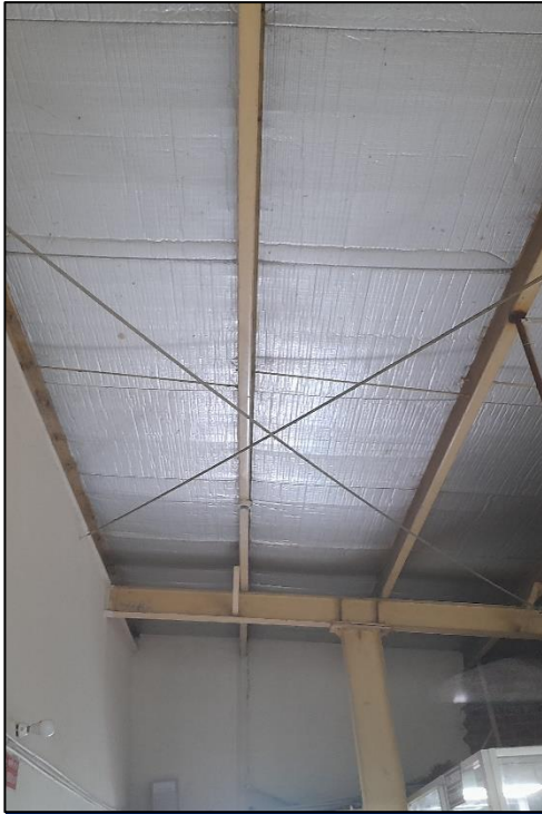
Roof & wall bracing provided
