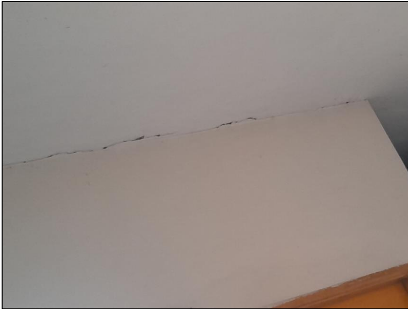
Cracks on masonry walls
